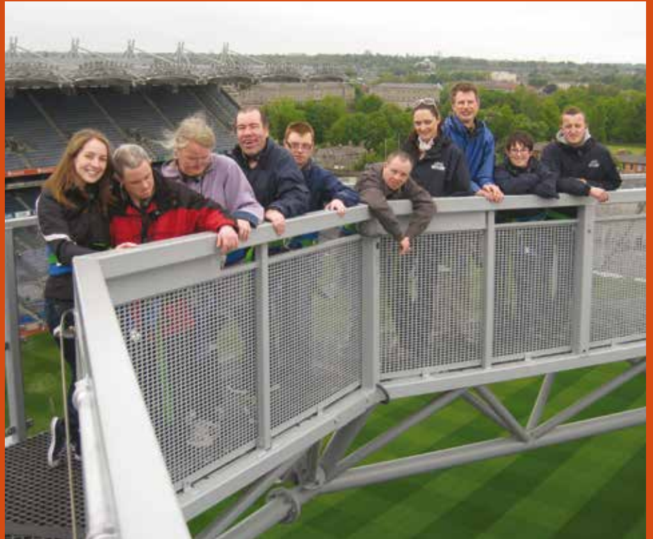
Bridge over the Park
